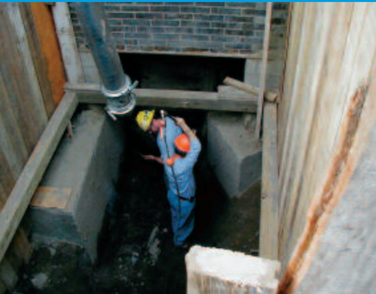
Repairing Steam Line under Foundation
