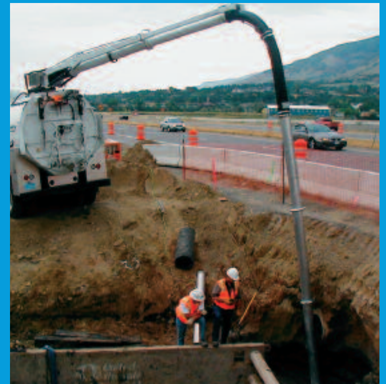
Drilling Mud Removal
