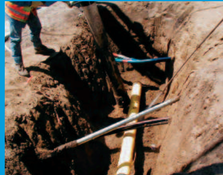
Multiple Utility Lines Safely Exposed
