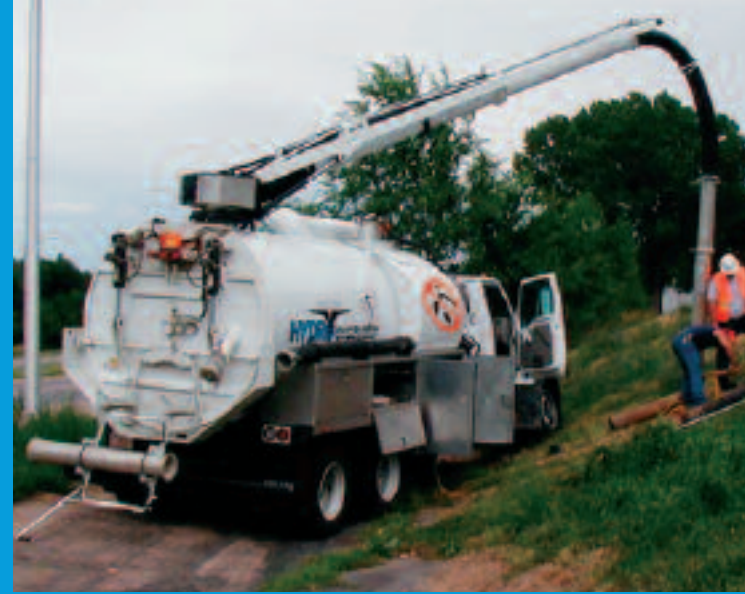
Water Shutoff Repair
